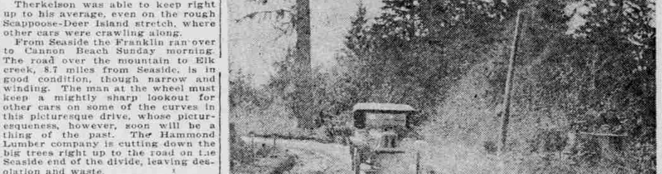
These views show how all but a narrow strip of macadam has been dug up for several miles on the lower Columbia river highway on the stretch between Clatskanie and Stevenson, preparatory to laying rock and hot stuff. In wet weather you are out of luck if you drop off the macadam in the center. Three paving plants have been set up between Clatskanie and Astoria and will soon be going full blast. The car in the picture is a Franklin.
