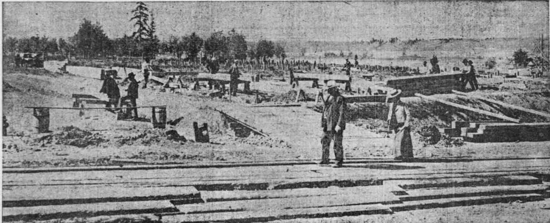
FOUNDATIONS OF LIBERAL ARTS BUILDING.
