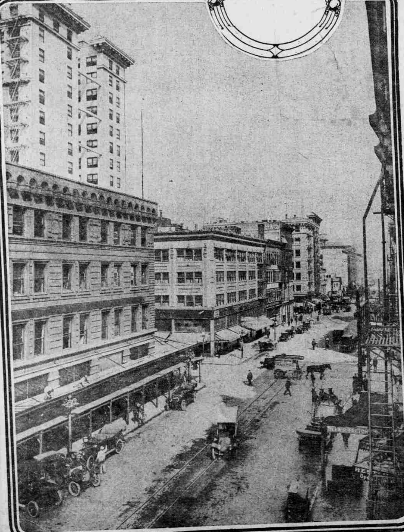
Fourth Street North From Alder
