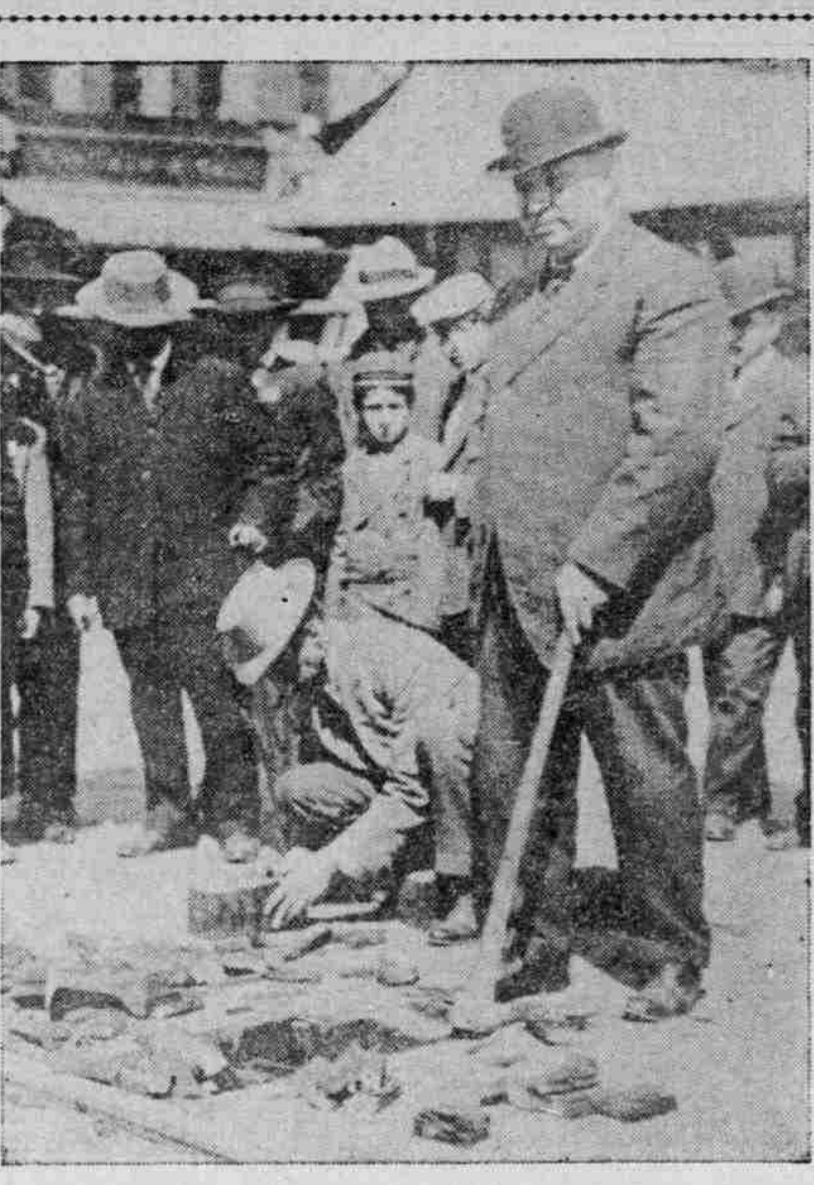
COUNCILMAN L. B. HOWARD, OF LEWISTON, EXAMINING WOOD-BLOCK PAVEMENT.
