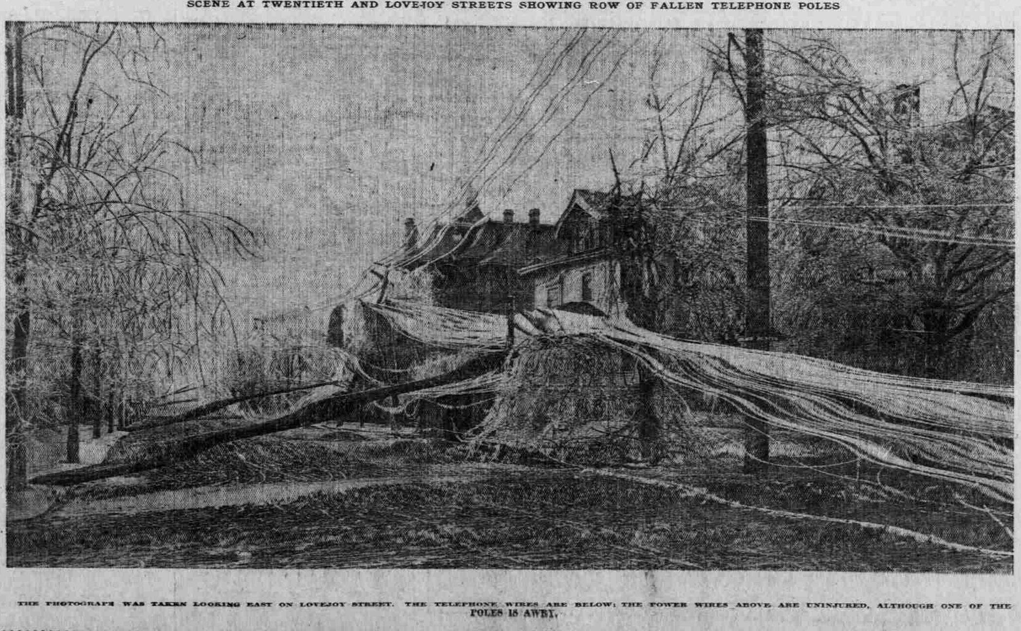
SCENE AT TWENTIETH AND LOVEJOY STREETS SHOWING ROW OF FALLEN TELEPHONE POLES
