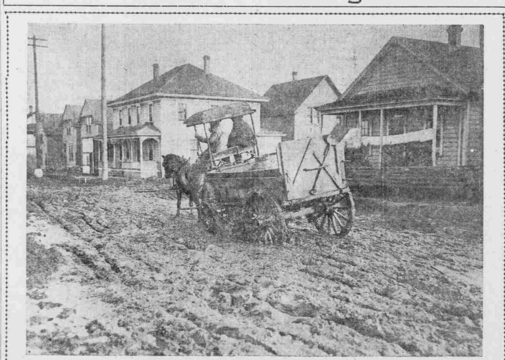
NICOLAI STREET MUDHOLE, OF WHICH SCAVENGERS COMPLAINED.
