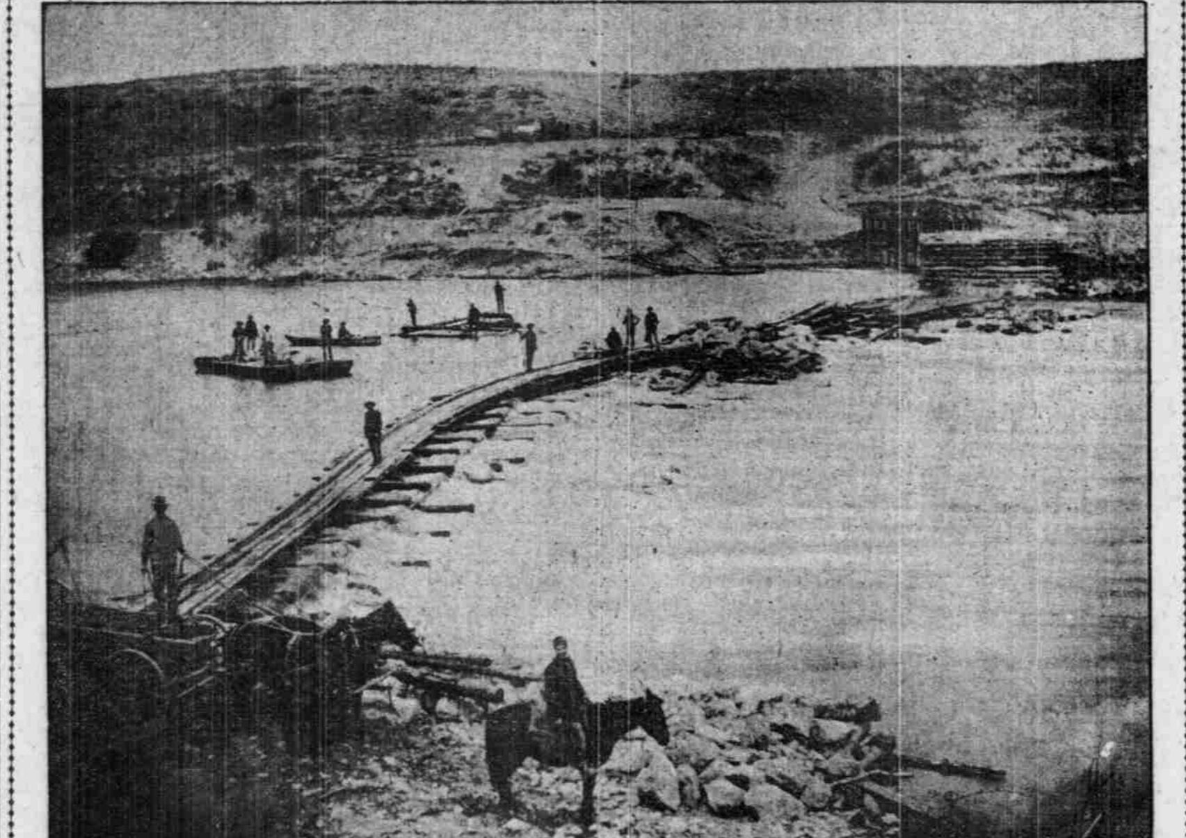
DAM TO TURN WATER FROM SNAKE RIVER INTO IRRIGATING CANAL AT IDAHO FALLS.
