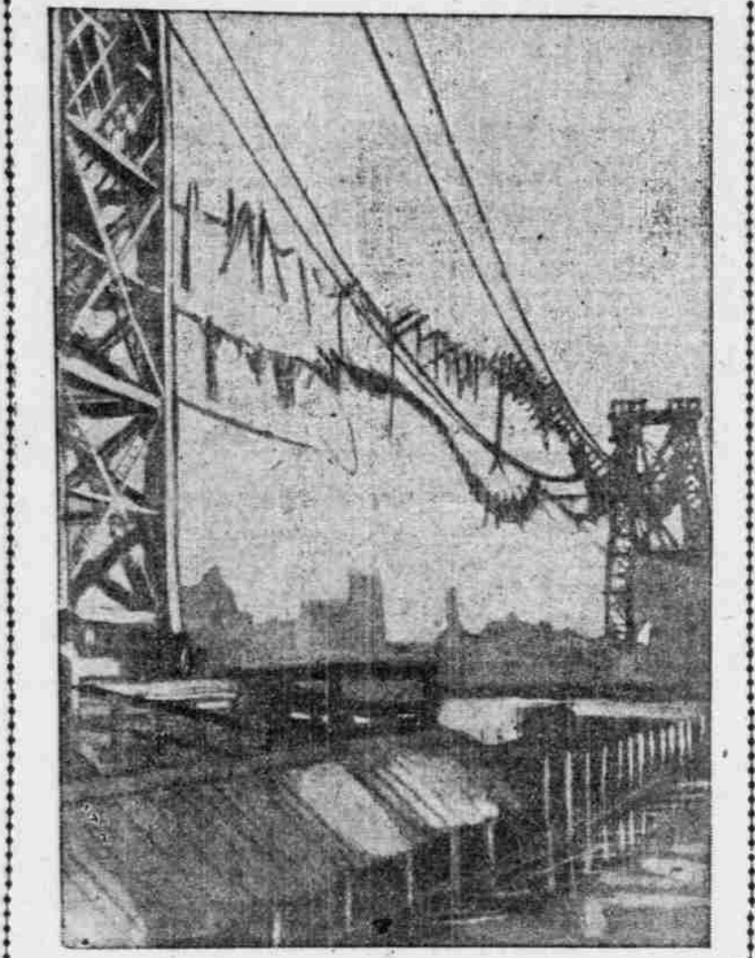
Damage to the extent of $50,000 and a further delay of two months seem to be the proper estimate for the fire in the west tower of the East River bridge. Detectives representing Fire Marshal Press made an investigation into the fire, and learned that it was caused by a workman who threw a lighted match on some inflammable material.
