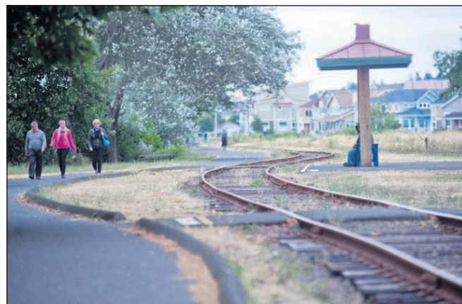
The city of Astoria acquired the right-of-way to a former Burlington Northern Santa Fe LLC rail corridor in 1996 through a railbanking agreement to preserve historic tracks.
