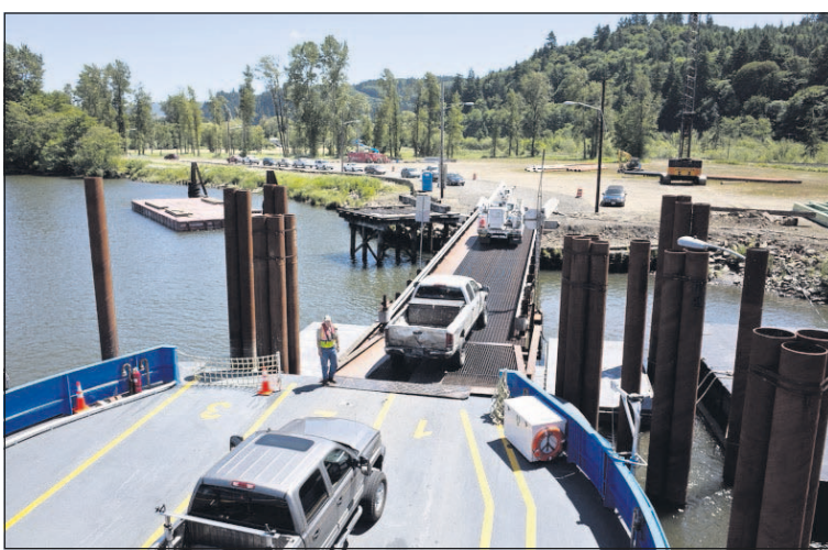
Cars exit the Oscar B as a line of cars wait to board at the dock in Westport. It takes about 15 minutes to cross the Columbia River on the ferry.
