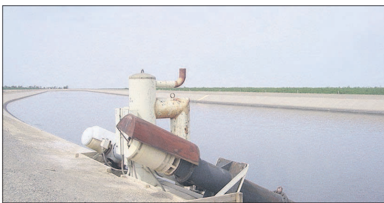
A pump takes water from a main canal south of Mendota, Calif., and sends it to a farm in this file photo. Growers on the west side of the San Joaquin Valley had their Central Valley Project allocation increased to 100 percent of requested supplies on April 11. Tim Hearden/Capital Press
